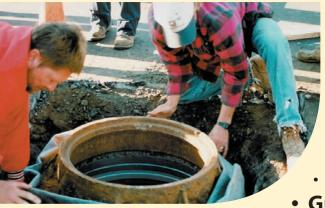
**Ladtech's** light weight adjusting rings are manufactured from 100% polyethylene recycled plastic. At approximately 6lbs., these rings are durable and provide for quick and easy installation.
