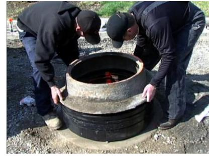
**11.** You will now proceed to install the cover frame. Prior to setting it in place, apply a 3/16 to 1/4 inch bead of the approved caulk butyl sealant or a 3/8 inch round rope ASTM C-990 on the top of the last ring. Be sure to apply the sealant in a location so that it contacts the cover frame the full 360 degrees. If necessary, you may apply a double bead of sealant.
