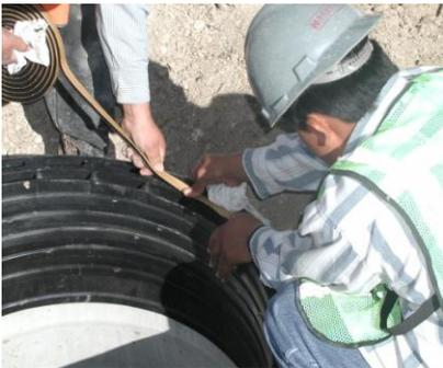
**12.** With the sealant applied, set the cover in place verifying that it is centered on the top ring.
