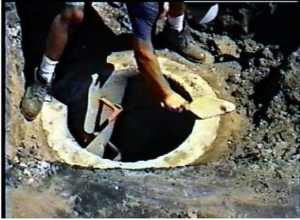
**1.** The first step is to make sure you have a clean installation area. Be sure to clean the concrete cone or top slab with a whisk broom or chisel. This will assure a flat seating surface free of rocks, gravel, blacktop, protruding concrete or frozen debris.
