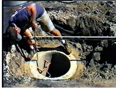
**2.** With the installation area now clean, measure the distance from the cone or top slab to the projected finish grade. When making this measurement, be sure to deduct the distance, or height, of the cover frame. Determine the net build-up of rings necessary to come within a 1/4 inch of the grade with the cover frame in place.
