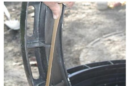
**8.** As before, place the second ring down onto the first with the male lip interlocking into the center of the first ring. For each ring, make sure to line up your paint strip.
