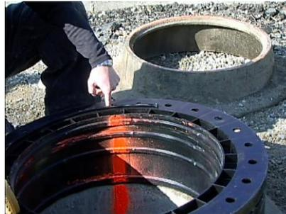
**5.** When the assembly is in place and you have your desired height and slope, mark the entire stack with a vertical line of spray-paint. Once you have your line, disassemble the set-up.
