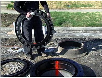
**9.** Repeat the assembly as you did in the prior steps for each additional ring, applying the bead of sealant and placing the rings on top of one another being sure to line up the paint strip.
