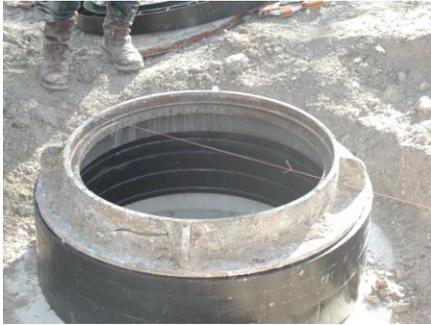
**4.** With the measurements determined and your required rings selected, dry stack the rings on the cone or top slab. Index any slope rings as necessary. With the rings dry-stacked, place the cover frame casting on top of the assembly and verify the height and slope match.
