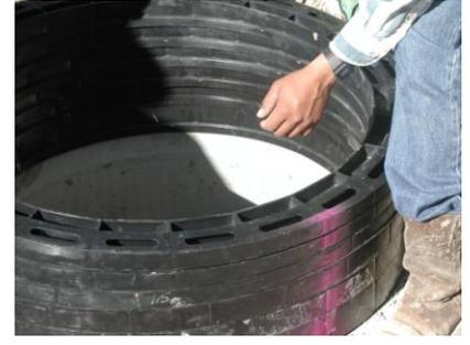
**3.** Now that you have your preliminary measurements, you will need to determine the best ring height combination to attain the necessary adjustment for your specific installation. In cases where grades are not flat, use slope rings to accommodate for this difference.
