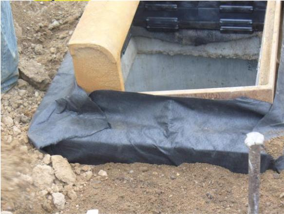
5. If the specifying engineer requires a woven, unwoven or poly fabric wrap, it should be applied at this time. If used, the wrap should extend over casting flange and a minimum of 4" below top edge of concrete structure. If oversize manhole with top slab, wrap should rest a minimum of 6" out from rings and on top of slab.
