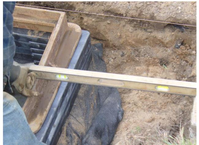
2. Stretch string line or position straightedge to determine height adjustment required.
