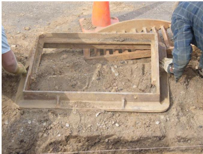
1. Remove existing casting and rings or cover plate to expose concrete structure.
