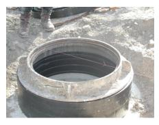
**4.** With the measurements determined and your required rings selected, dry stack the rings on the cone or top slab. Index any slope rings as necessary. With the rings dry-stacked, place the cover frame casting on top of the assembly and verify the height and slope match.
