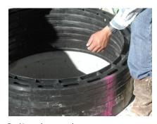
**3.** Now that you have your preliminary measurements, you will need to determine the best ring height combination to attain the necessary adjustment for your specific installation. In cases where grades are not flat, use slope rings to accommodate for this difference.
