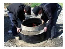
**11.** You will now proceed to install the cover frame. Prior to setting it in place, apply a 3/16 to 1/4 inch bead of the approved caulk butyl sealant or a 3/8 inch round rope ASTM C-990 on the top of the last ring. Be sure to apply the sealant in a location so that it contacts the cover frame the full 360 degrees. If necessary, you may apply a double bead of sealant.
