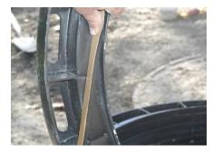
**8.** As before, place the second ring down onto the first with the male lip interlocking into the center of the first ring. For each ring, make sure to line up your paint strip.
