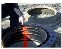
**5.** When the assembly is in place and you have your desired height and slope, mark the entire stack with a vertical line of spray-paint. Once you have your line, disassemble the set-up.
