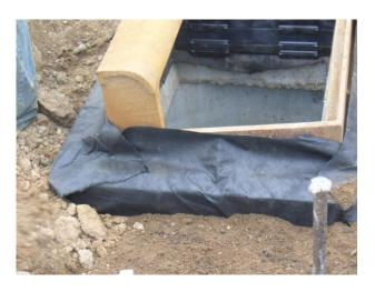
5. If the specifying engineer requires a woven, unwoven or poly fabric wrap, it should be applied at this time. If used, the wrap should extend over casting flange and a minimum of 4" below top edge of concrete structure. If oversize manhole with top slab, wrap should rest a minimum of 6" out from rings and on top of slab.
