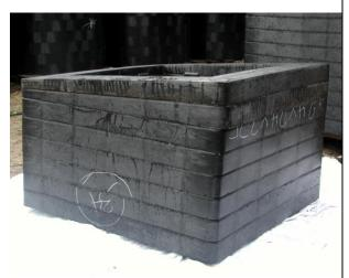
3. Combine various ring heights, in both flat and slope, to reach desired adjustment. Rings are to be placed with pocket openings down and tabs extending into structure or lower rings. Note: Slope rings are tapered from side to side at an angle to prove a 1% to 3% grade compensation.
