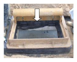
4. If offset of rings is needed to achieve casting-to-curb alignment, use a saw to remove interlocking tabs from underside of ring(s) as necessary. Removal of tabs from one side of end of ring will allow up to 2 " of offset. Offset should not exceed this amount per ring. Removal of tabs from more than one side will allow for rotation of the rings. Note: Total offset of all rings should not exceed 4" without a concrete collar being poured to maintain stability and integrity of structure.
