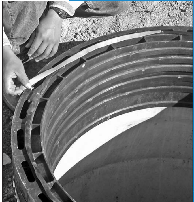
Photo: Worker installing butyl rubber rope
